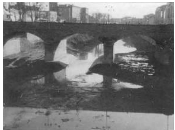
Mathew Bridge before rewatering
