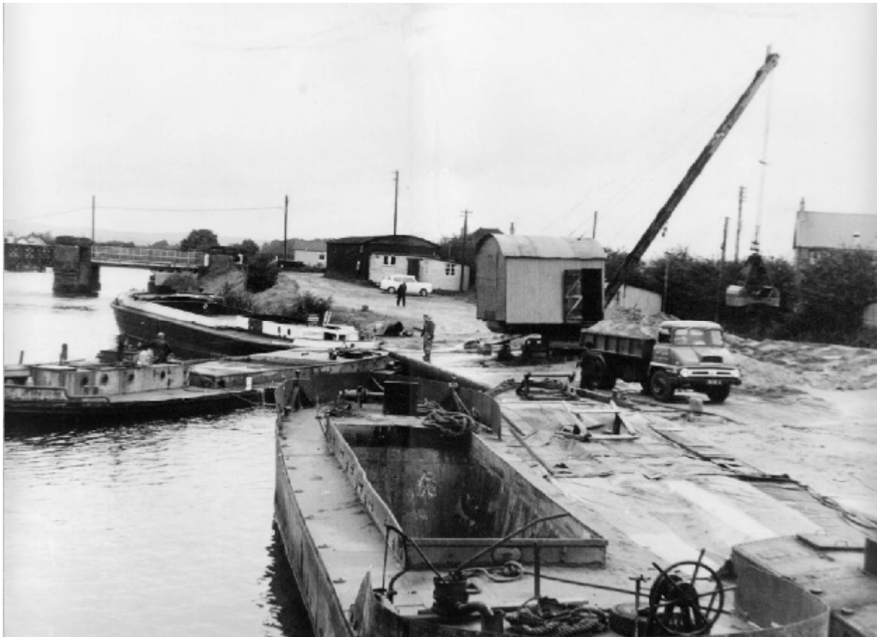
Clonsilla waiting to unload and Killiney behind being fitted out for sand dredging
