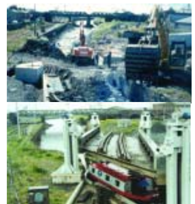
Before and after: work on the Royal
